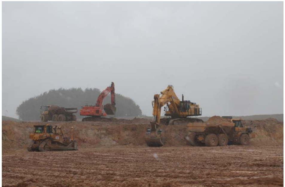
Figure 15: Shovel and ore loading operations in the Drakelands pit
