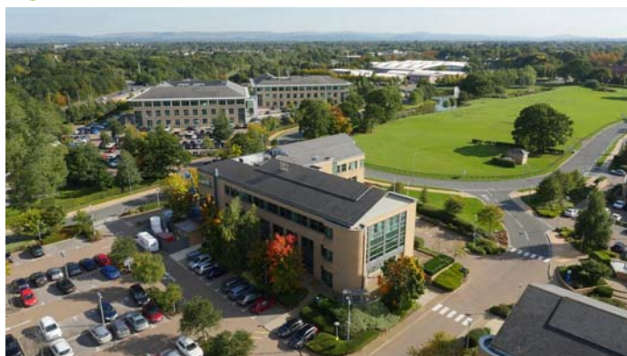
Figure 20: Lakeside 5500 - exterior aerial
