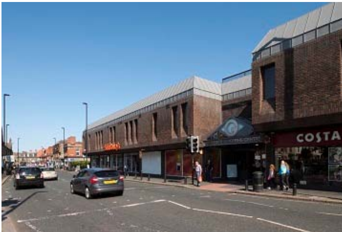
Figure 15: Gosforth Shopping Centre - exterior
