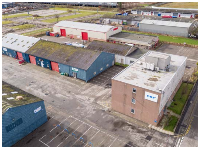
Figure 5: Burnside Industrial Estate, Aberdeen - exterior
