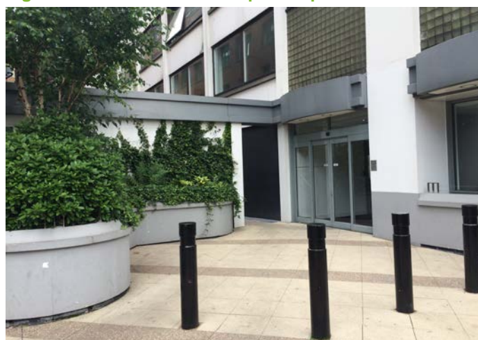
Figure 15: Arthur House reception – previous exterior
