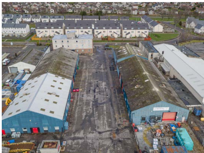
Figure 4: Burnside Industrial Estate, Aberdeen - exterior
