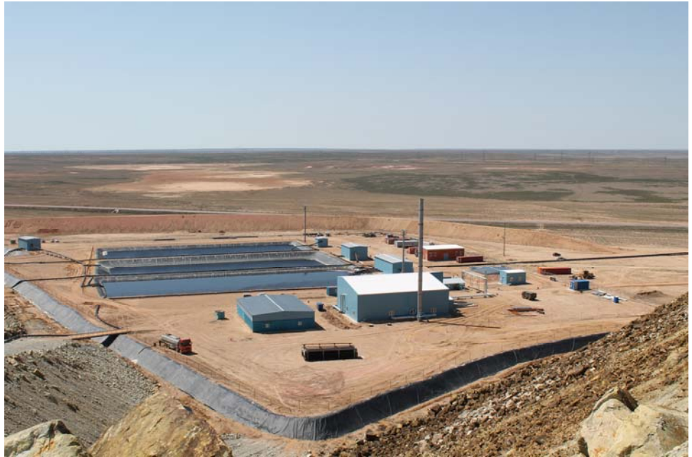
Figure 11: The new collection, boiler and pumping infrastructure for the Western dumps
