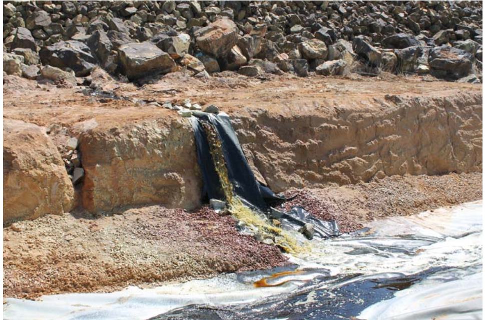
Figure 10: PLS pouring into the collector trench from the ILA
