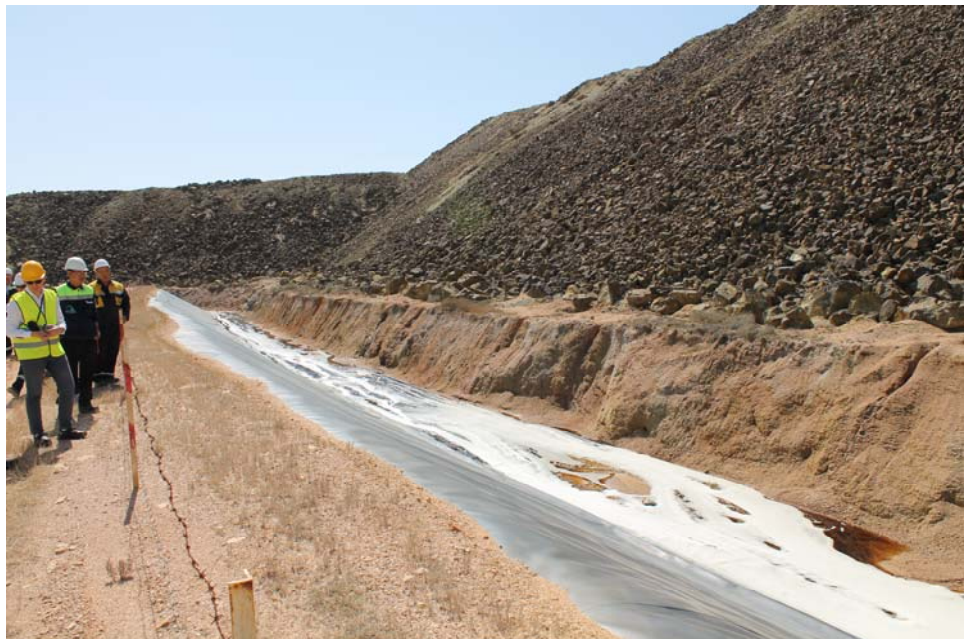
Figure 5: PLS collection trench at the bottom of the Eastern dumps
